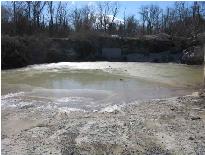
Truck Wash-out Basin
