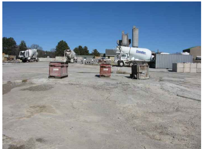
Barrier Block Manufacturing Area and Run-off Area to Outfall 001
