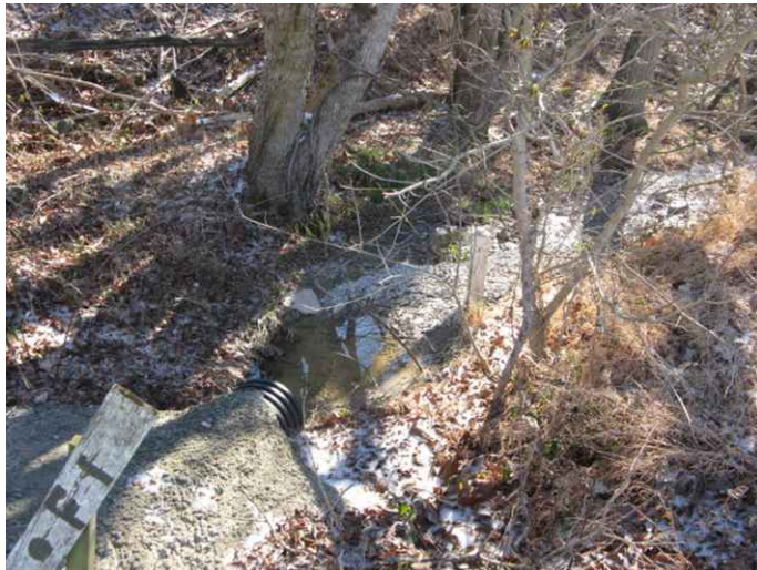
Outfall 001 Receiving Channel
